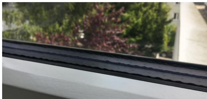
Image 01: Butyl reaching into the cavity
